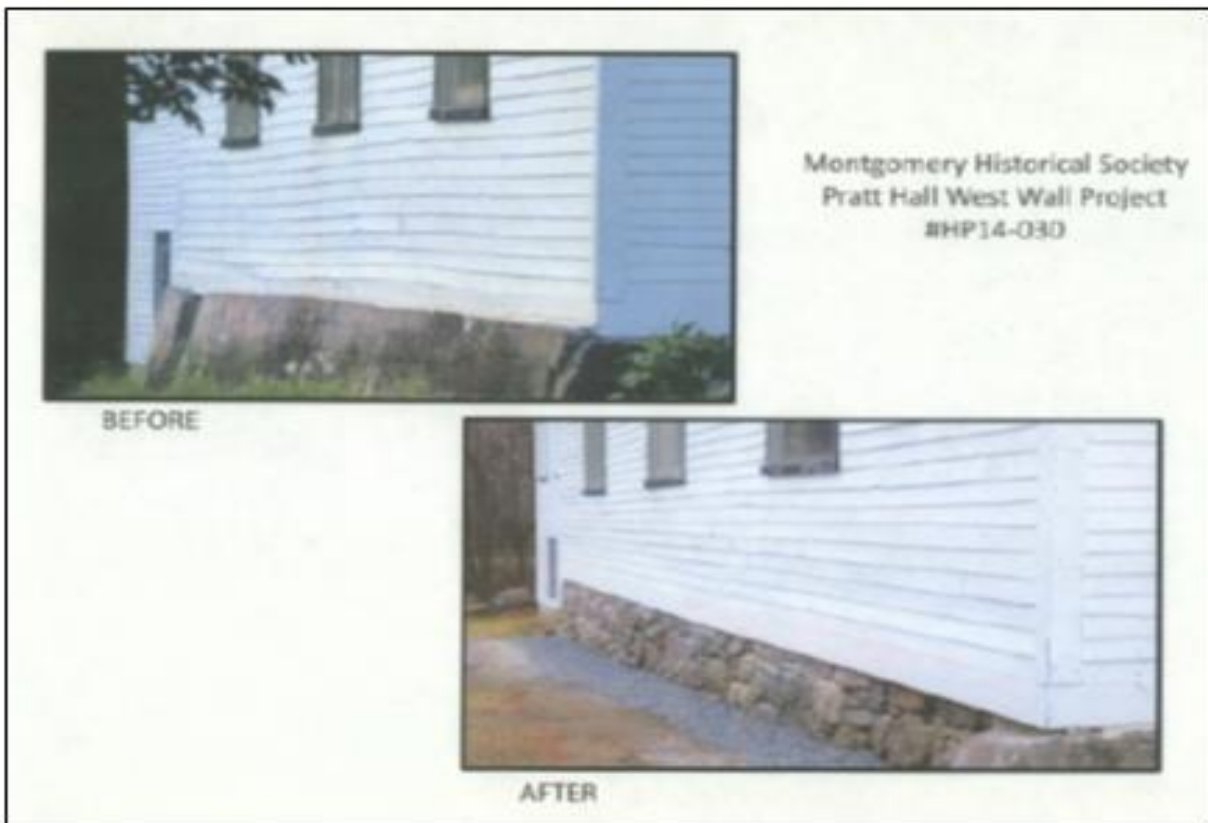
Pratt Hall, Montgomery $20,000 for structural and foundation repairs to the west wall
